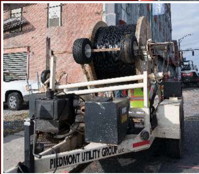
Fiber optic cable waiting to be pulled into the building
