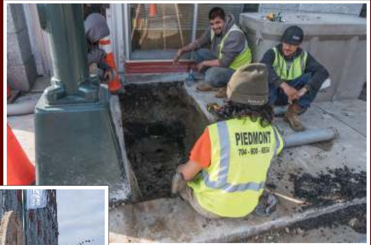
Ready for the new hand hole box
